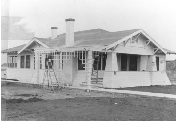
Construction of a Bungalow Colony unit, 1920. Source unknown.
