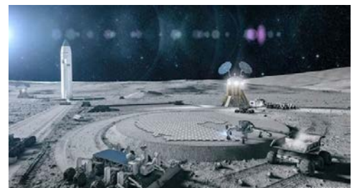
Rendering of what the early phases of a colony on the Moon might look like. In the foreground, robots are building a launch pad with bricks created by grinding, melting and re-shaping basaltic moon rocks. (Image courtesy of XArc)
